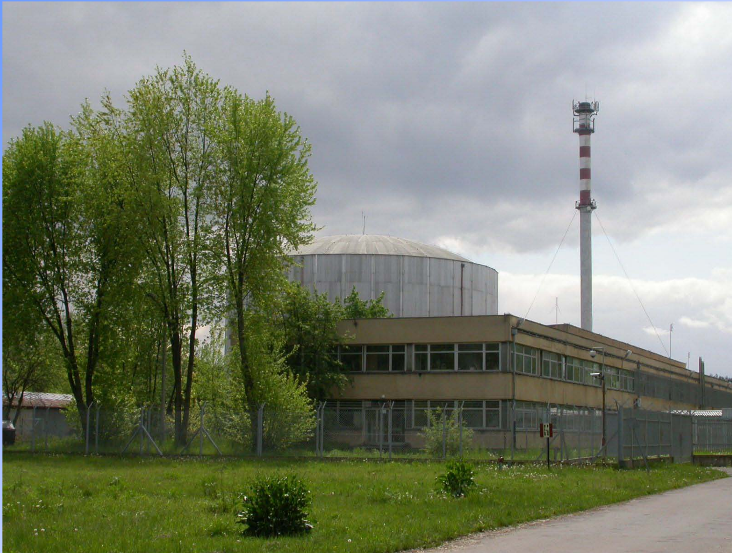
General view of MARIA reactor
